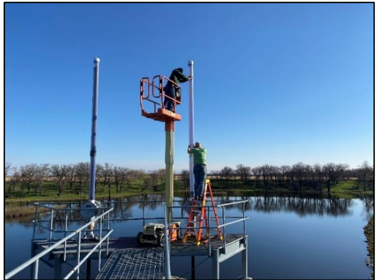
Gate stem covers after replacement.
