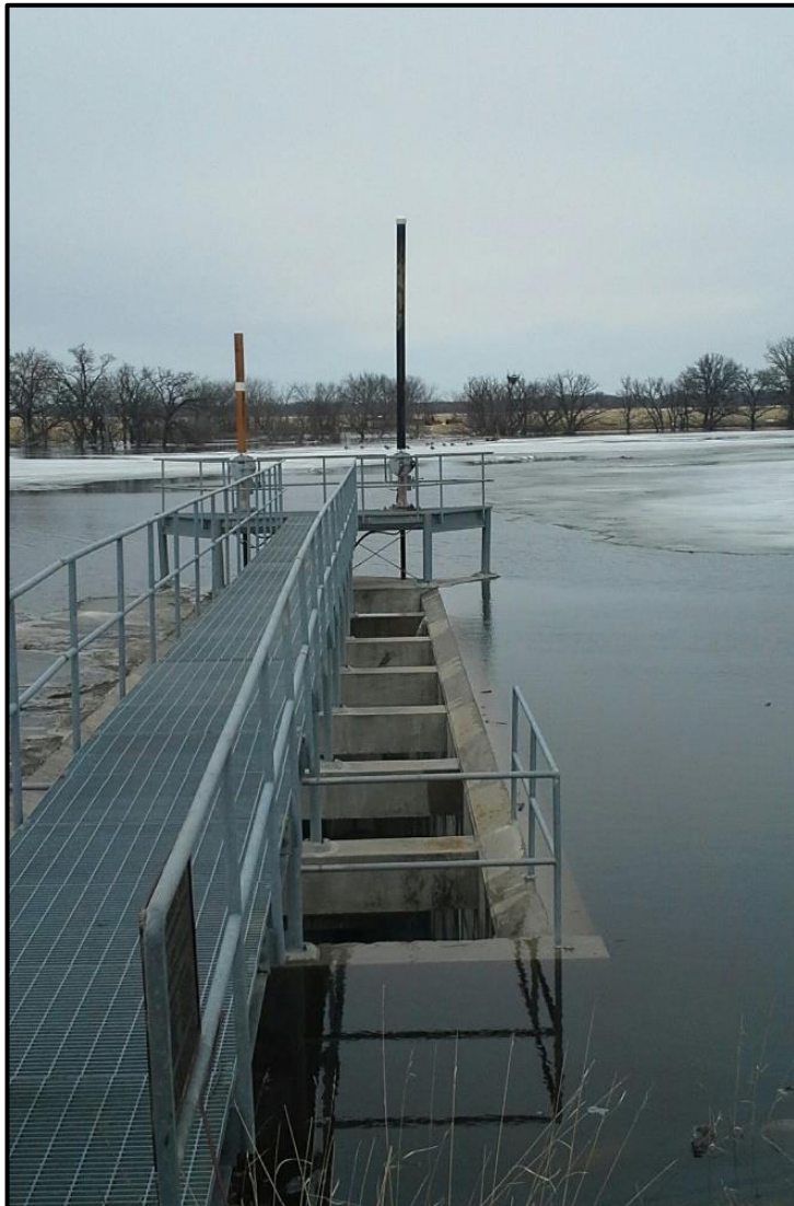
Gate stem covers after replacement.
