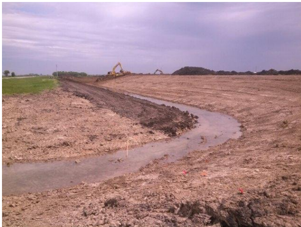
Ditch along TH #220 looking south
