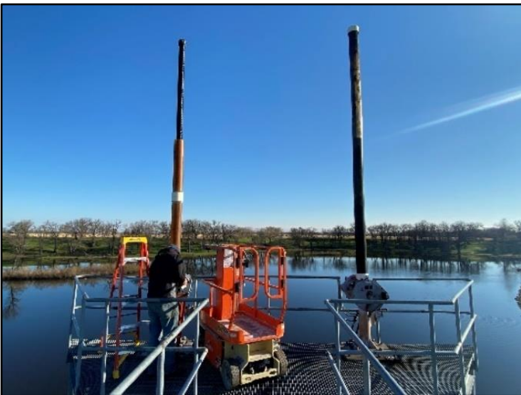
Gate stem covers after replacement.
