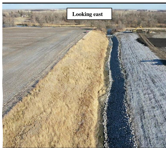
Bank Stabilization Project, Outlet of Pennington County Ditch 96 Pennington County SWCD
