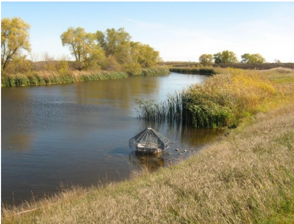
Latendresse Dam located in Red Lake Falls Township, Red Lake County
