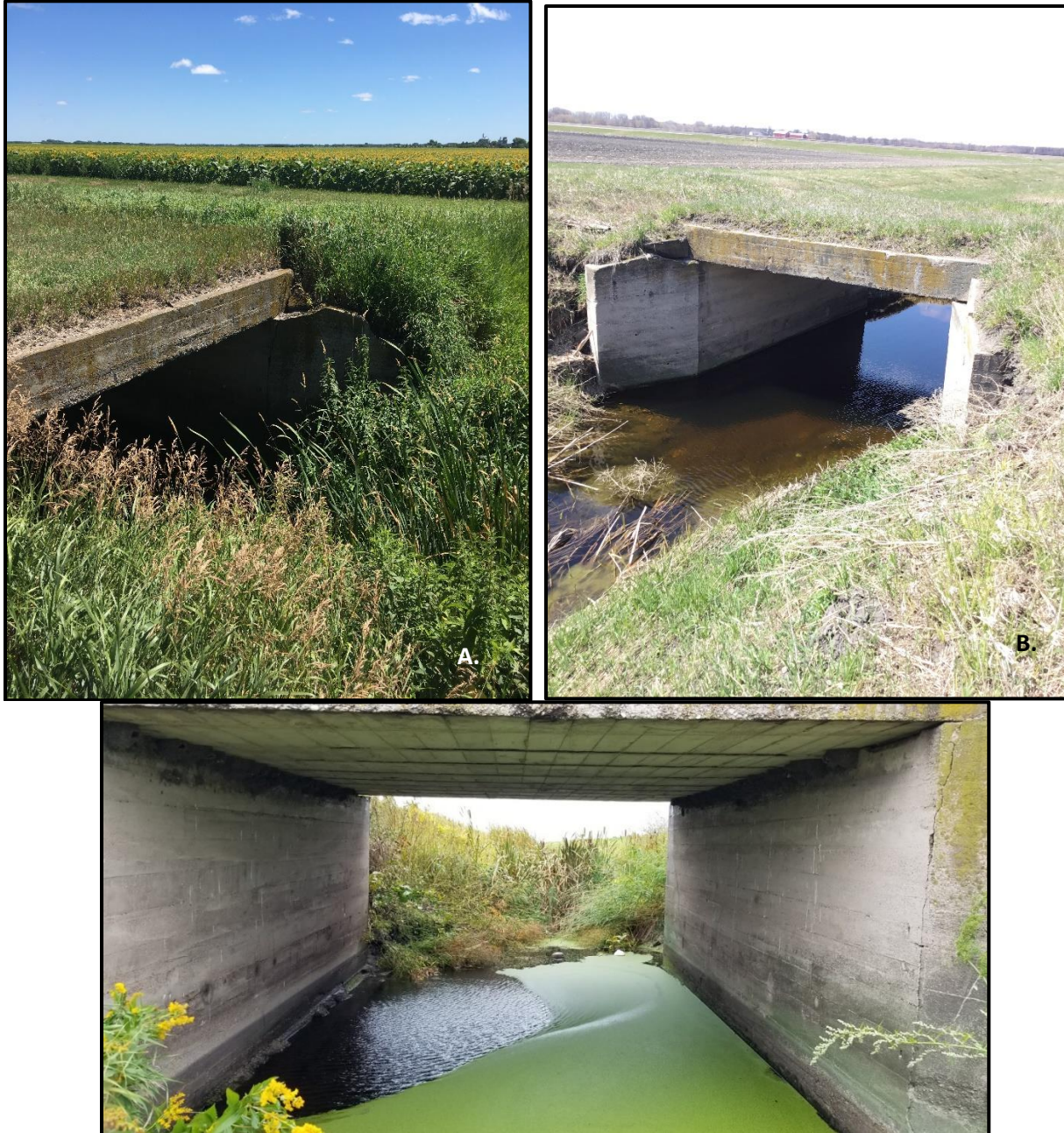
A. South west corner of failing bridge. B. East side of failing bridge. C. Under failing bridge, looking west.
